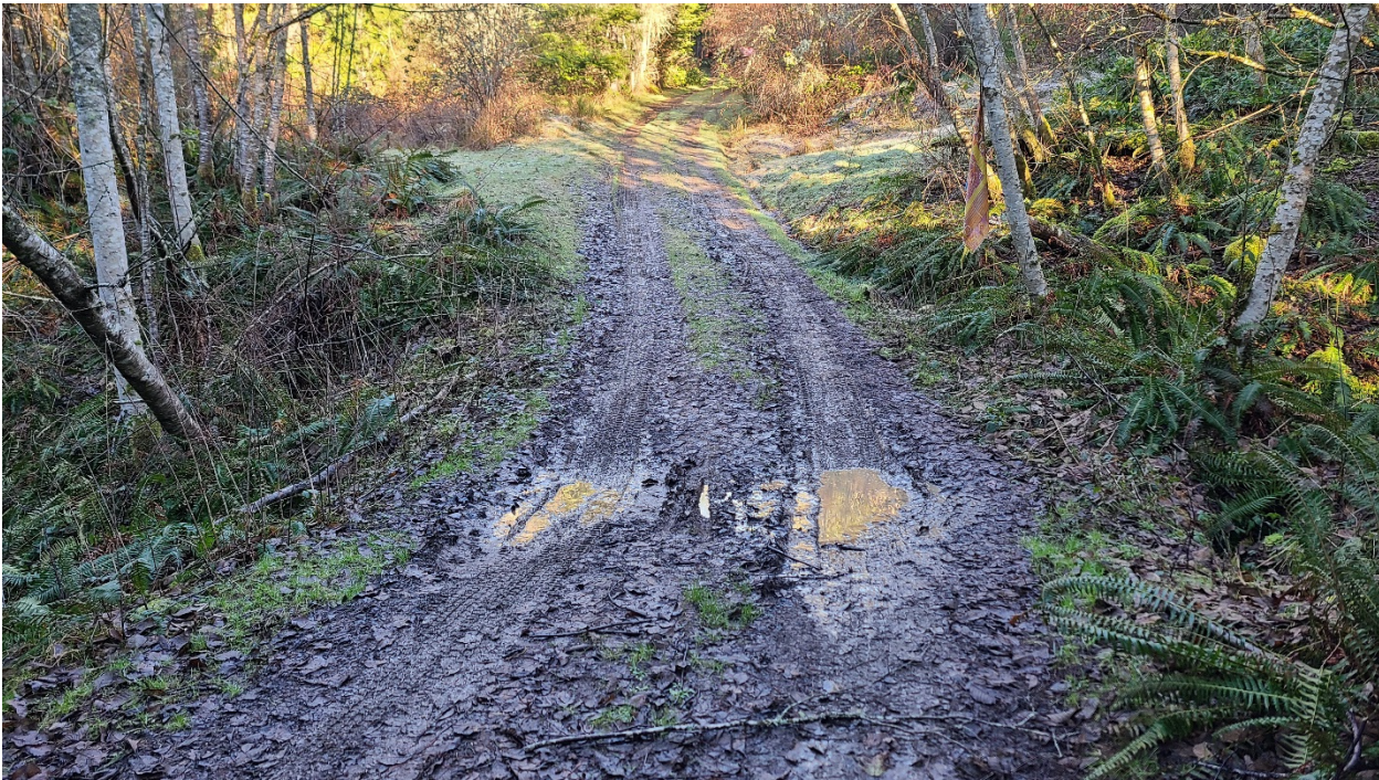
Photo 7 Emergency access road to be transferred to ITC
